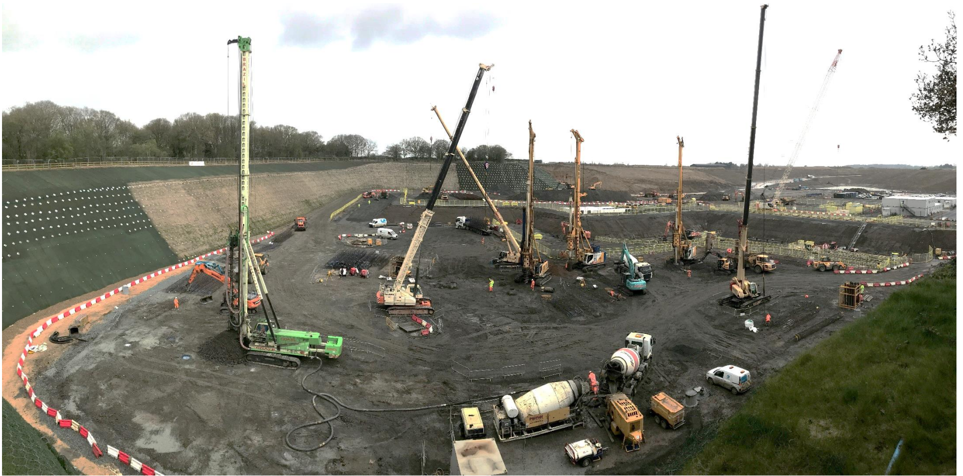
Figure 2.1: Excavation, soil nailing and piling works of the Consented Scheme
