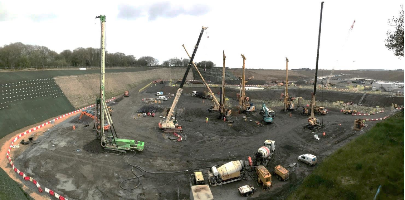
Figure 2.3: Excavation, soil nailing and piling works of the Consented Scheme
